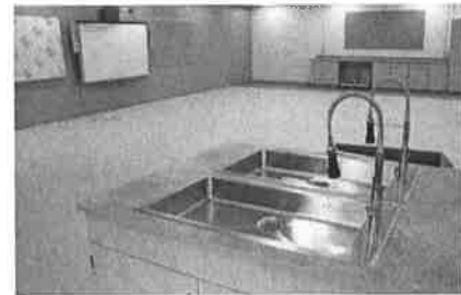
The renovated art room has new sinks and a new storage area.
