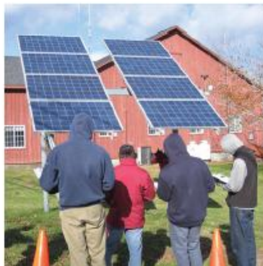
Photo 1—Small PV array with eight modules produces 1,840 W.
